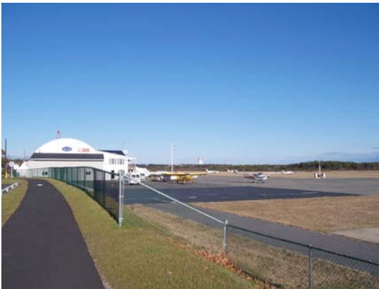
Figure 2.7-3: Chatham Municipal Airport
